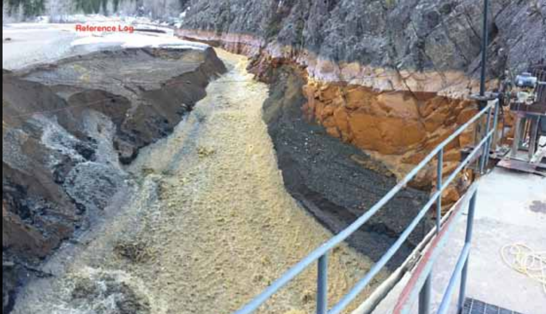
Sediment release flowing out of the Ouray Hydrodam reservoir Photo by Agnieszka Przeszlowska
