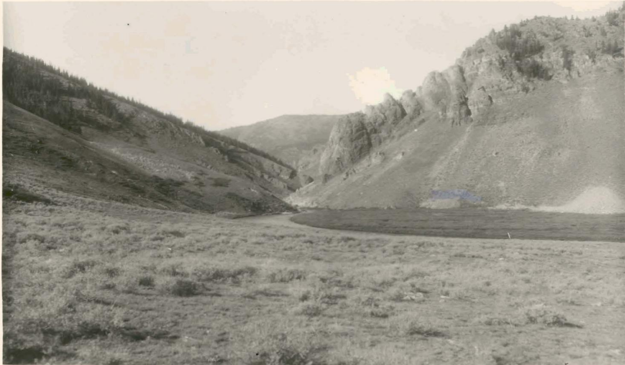
Taylor Park Dam Site
